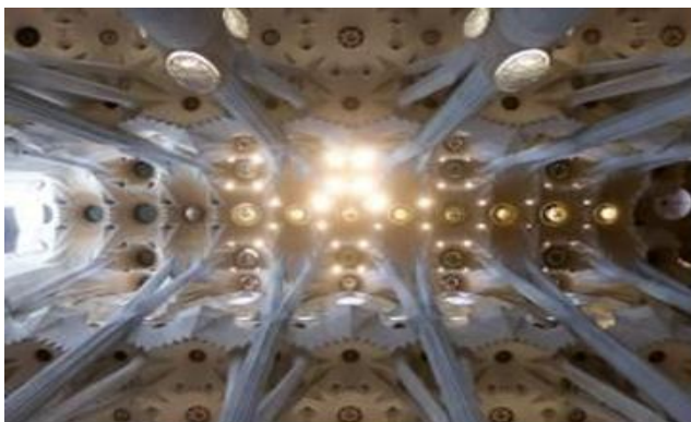
Figure 2: Gaudi used skylights among the columns, for bringing light into the building. Photo: TimBray Commons (Giuffo, 2011)
