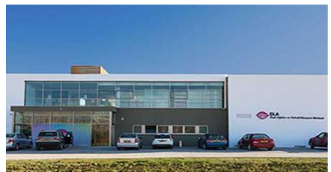
Figure1: Building Façade which is rectangular form has neutral and pastel color schemes (Taheri, et al., 2017)
